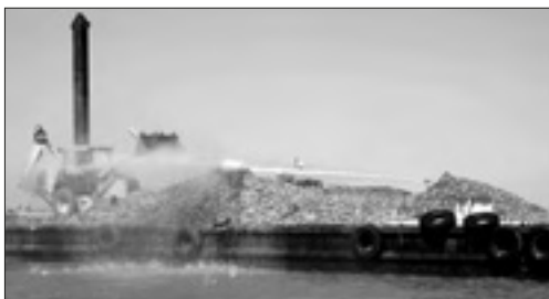
RESTORING THE REEF: Oyster shells are blown into Copano Bay from a barge in The Nature Conservancy's oyster-reef restoration pilot project. Photo by Mark Dumesnil, The Nature Conservancy.
