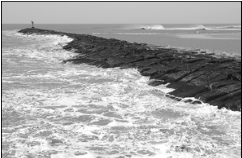
SHALLOW RUN: The Matagorda east jetty is angled, and silt has collected in the basin west of this jetty. A new jetty will be built parallel to the west jetty. Photo by David J. Sams, LSON.
